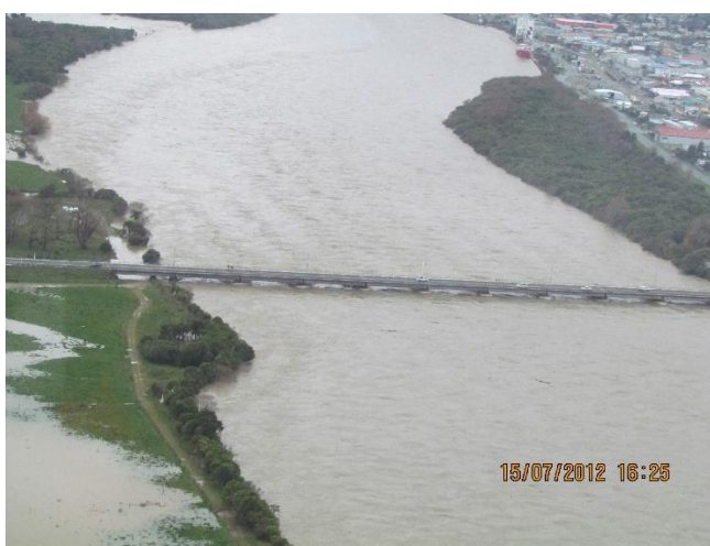
Figure 3-1 – Flood level at Buller River Bridge
