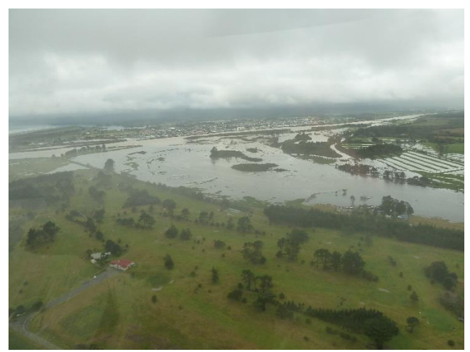
Figure 3-2 – Flooding on true left bank
