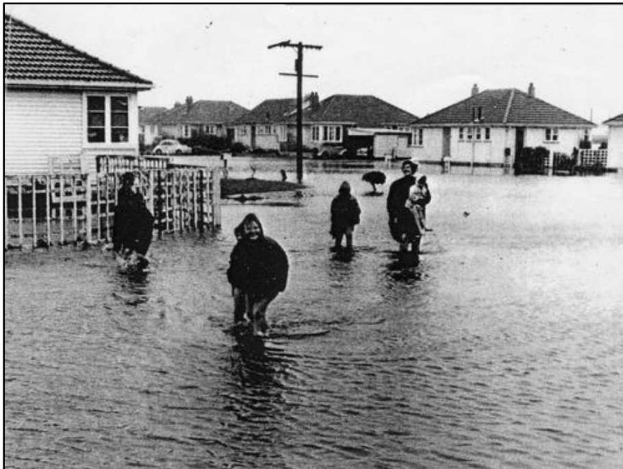
Figure 1-3 – Floodwaters in Westport during the 1970 flood event (Duncan, 2003)
