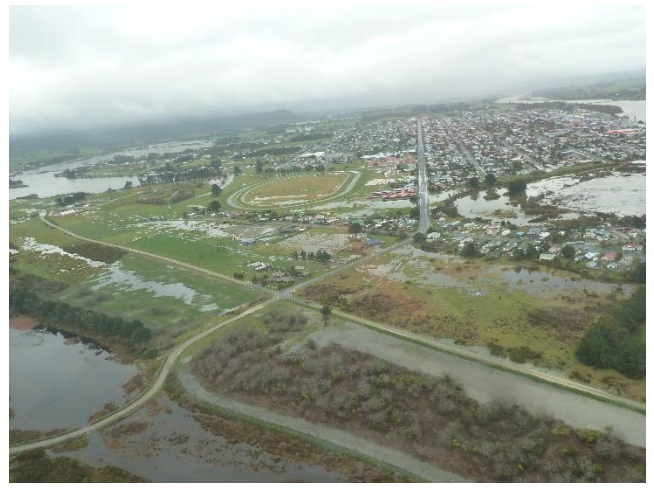
Figure 3-4 - Flooding in Westport Town
