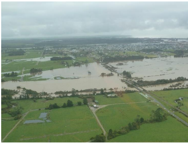
Figure 3-3 - Orowaiti Lagoon flooding
